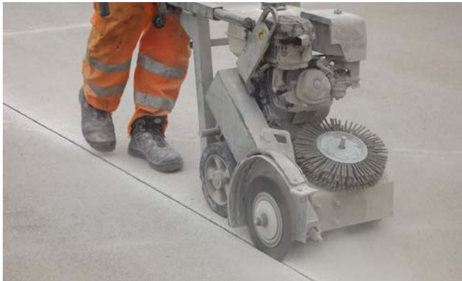
Joint brush used in road construction.
